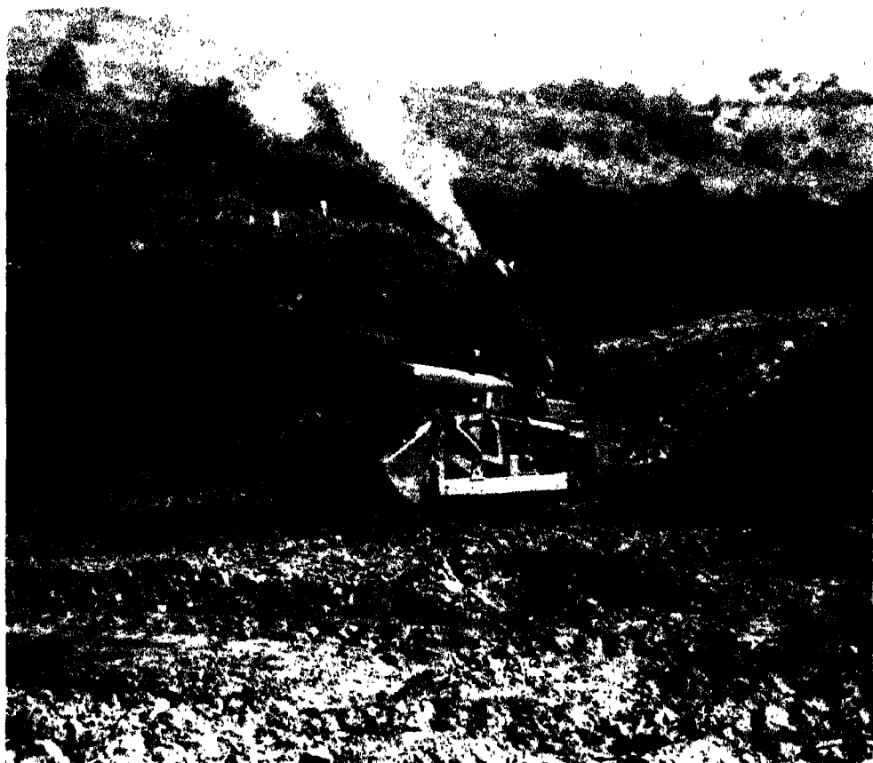
PLATE 7. Pond basin being cleared of brush by bull-dozing and burning (upper center). "Clam-dozer" removing sod to one side in foreground. This machine combines the advantages of the bull-dozer and power shovel with its hydraulically-controlled bucket-blade on front
