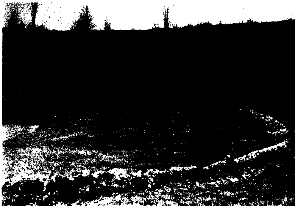
PLATE 14. A diversion ditch (terrace) is often useful to carry excess surface water away from the pond. The one shown is newly plowed, will be smoothed over and seeded to a grass sod.
