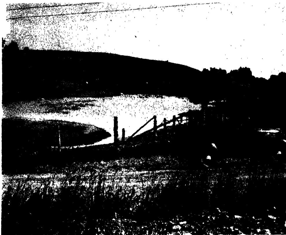
PLATE 12. Emergency spillway carrying off flood water after very hard rain Had the spillway not been there the dam would have been lost.
