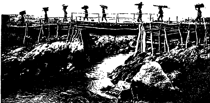
A BRIDGE ON THE HIGHWAY
