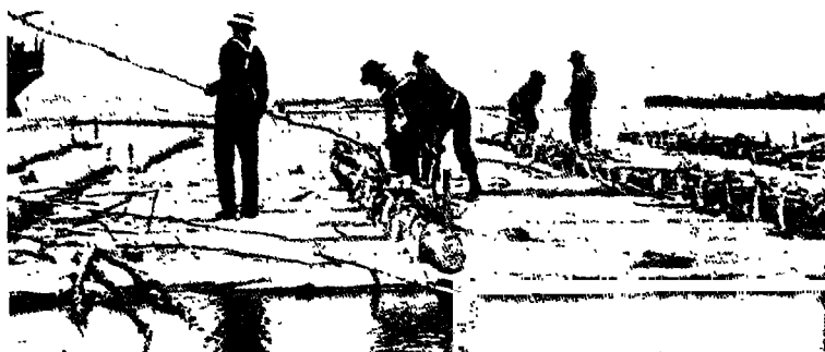
CONSTRUCTING A SQUARE-TIMBER RAFT
