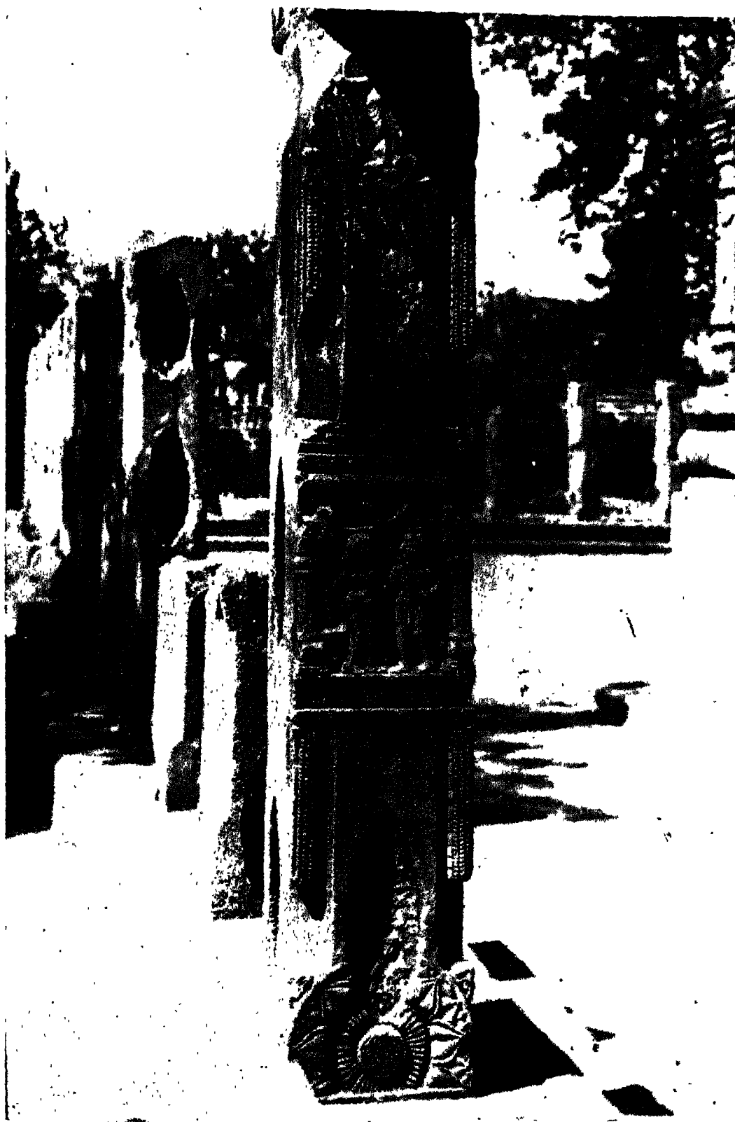
Fig. 15. A SOUTH-WEST CORNER VIEW OF PRESENT RAILING.
