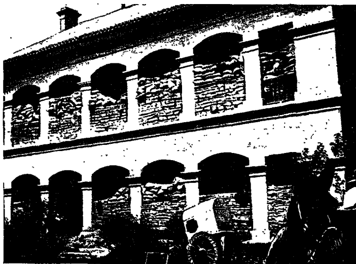
A SANDBAGGED HOUSE IN THE BRITISH LEGATION
