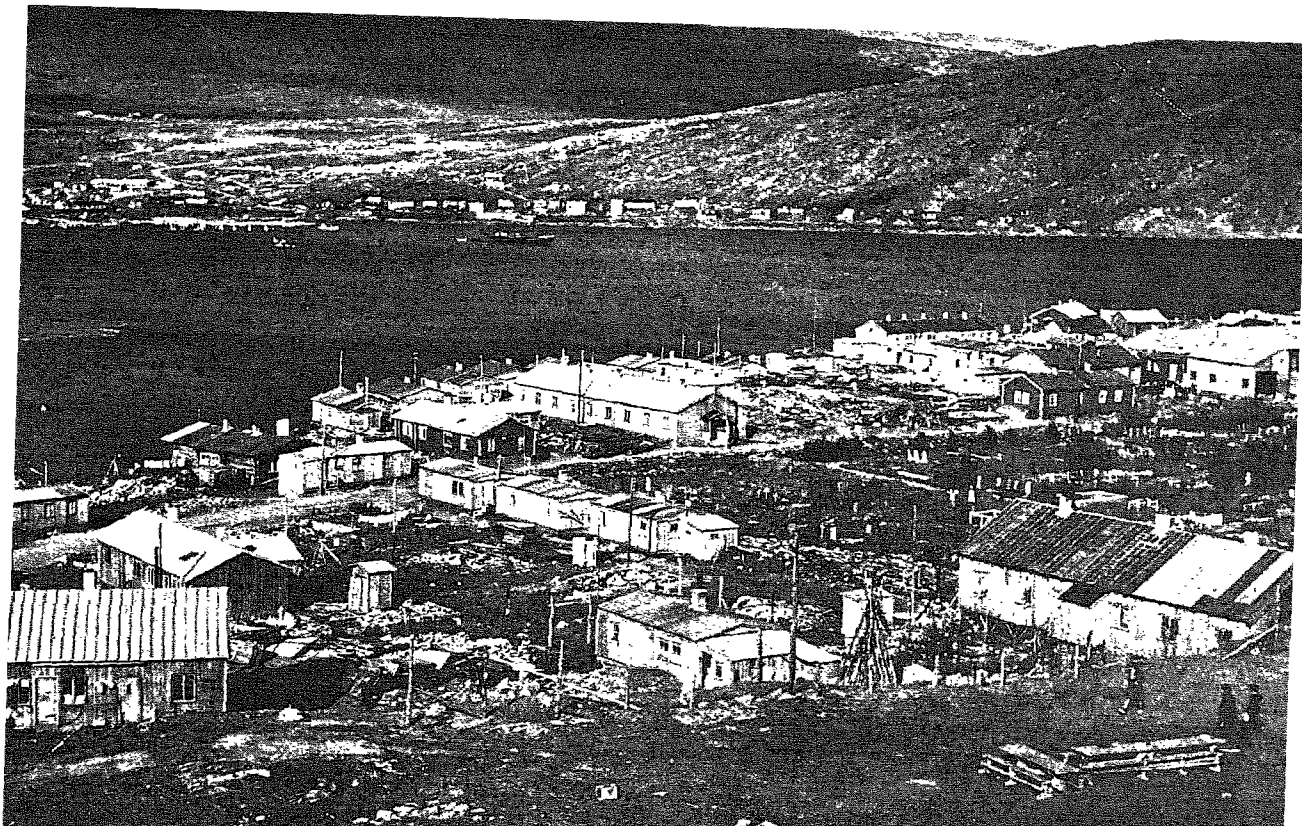
evastated Hammerfest under reconstruction.
