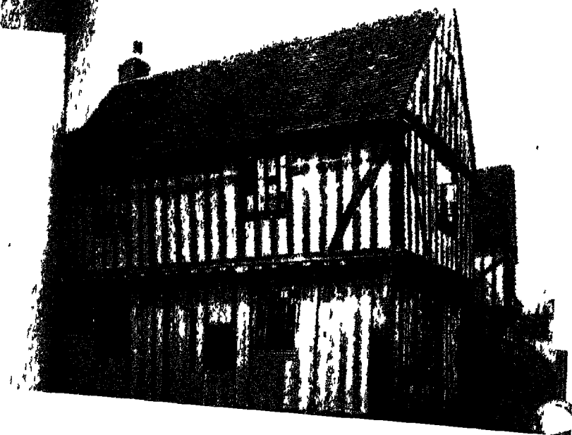
§112 The Wool Hall, Lavenham, Suffolk
