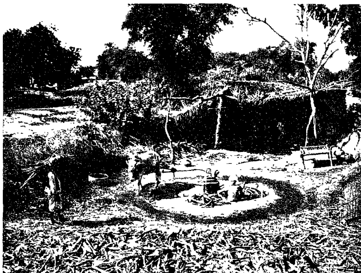
CATTLE AT WORK Crushing sugar-cane by bullock-power. (By the size of the cane it appears to be a superior quality, as also does the bullock. The machine is the old kolhu , now generally replaced by iron three-roller mills.) (See Chapter V, para. 19.)
