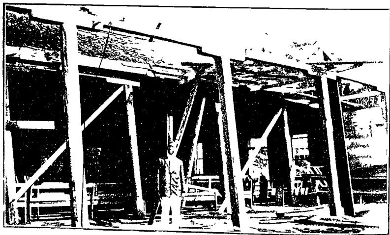
CYCLONE WRECKAGE SHOKWOOD CHURCH (THE INTERIOR)
