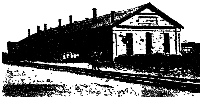
TIENSIN RAILWAY STATION SHELL D
