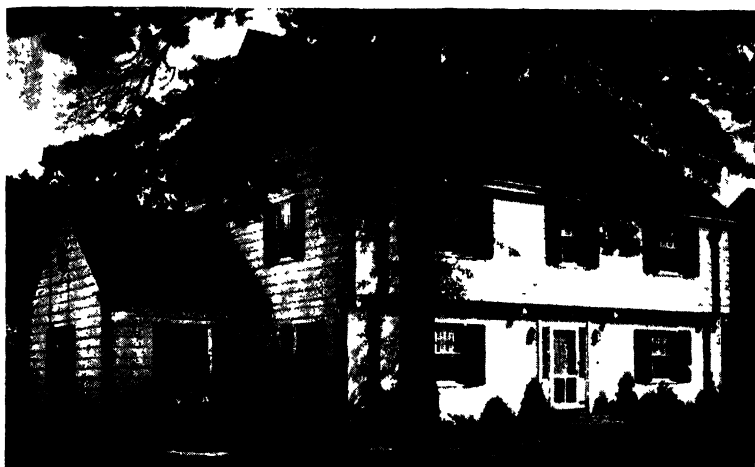
Fig. 8. Garrison Colonial House
