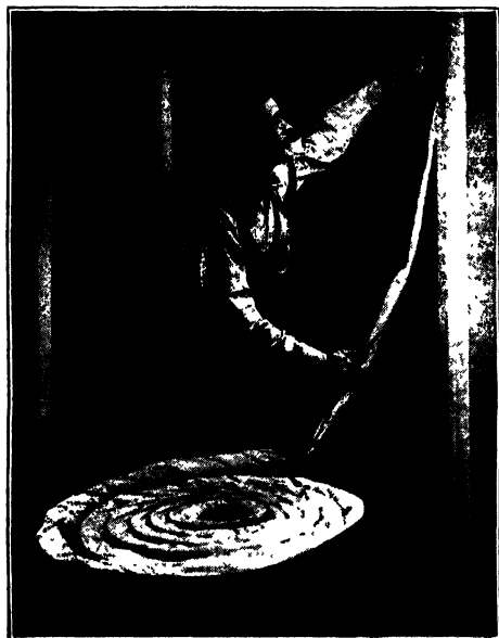
Fig. 164. How Typical Blanket Insulation Is Placed Between Studs
