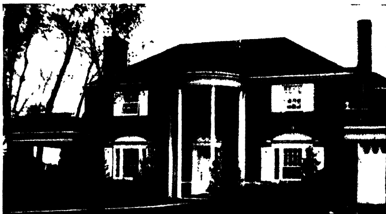
Fig. 13. Southern Colonial Style House
