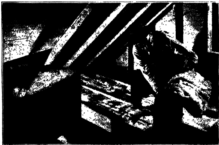
Fig. 163. How Typical Blanket Insulation Is Placed Between Attic-Floor Joists Courtesy of U.S. Gypsum Company, Chicago, Ill.
