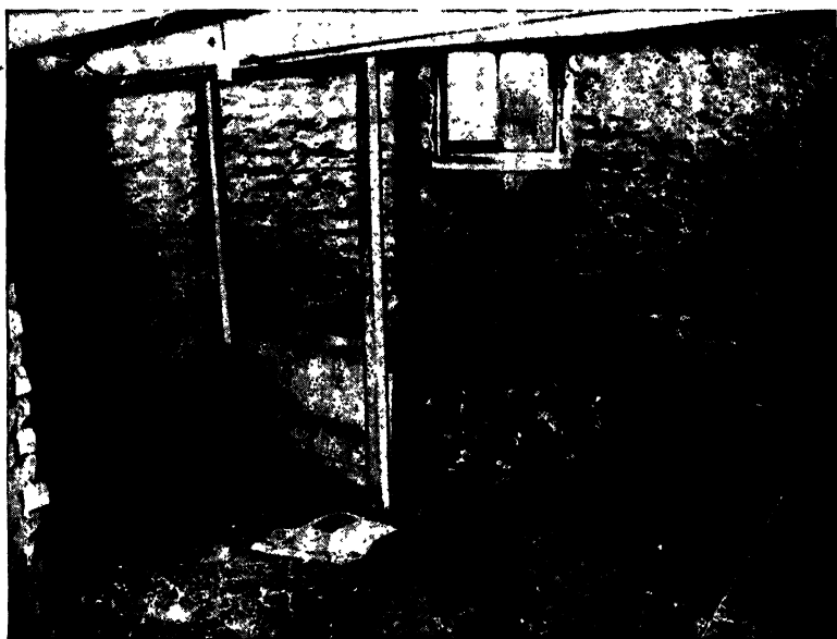
Fig. 306. View in Basement of Old House Showing Masonry Walls and Cracked Concrete Floor
