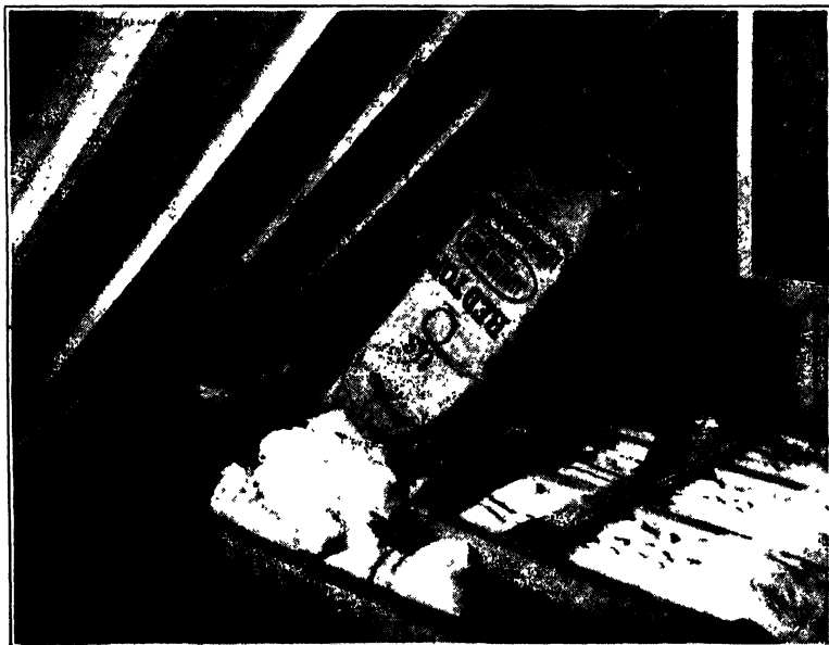
Fig. 151. Type of Fill Insulation Courtesy of U. S. Gypsum Company, Chicago, Ill.
