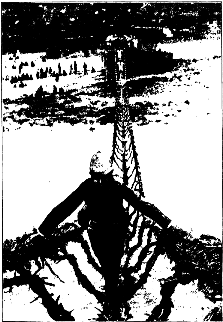
CROSSING A ROPE BRIDGE.
