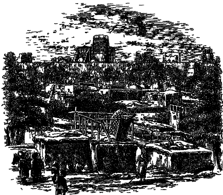
A VIEW INSIDE THE EXTERIOR WALL.
